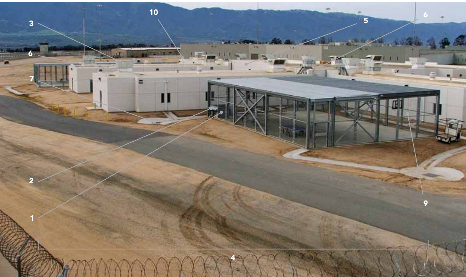
At the Salinas Valley State Prison in California, fixtures from Acorn Engineering Co., together with AcornVac® and Master-Trol® technologies, boost security and efficiency while conserving water.
